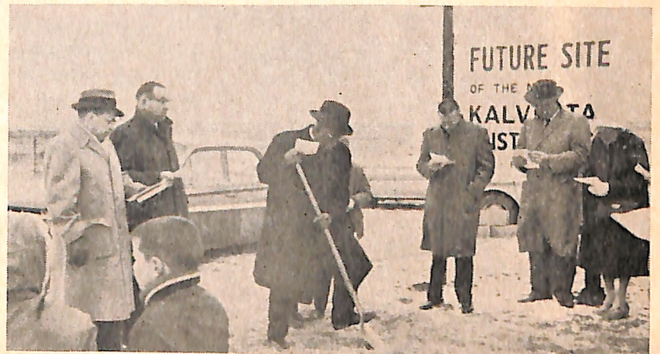
Clair, Jr., and Kalvesta Methodists from breaking ground February 10 for a $40,000 church building. The 80-member congregation is led by the Rev. William Wilkoff and Hayes Baldwin.
